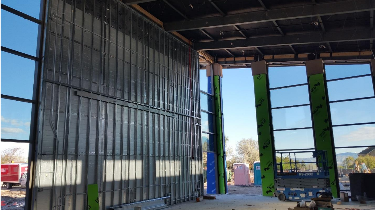
West wall of the Multi-purpose room before gypsum board is installed
