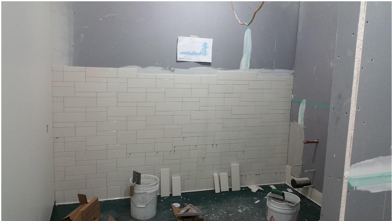
Bathroom wall tile is being installed in police area
