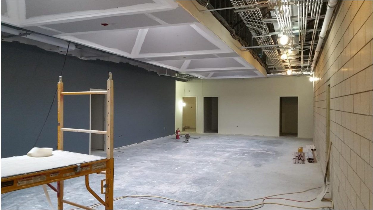
Sergents area walls are now painted
