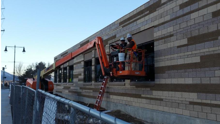
*Window frames and glass being installed on East side of City Hall*
