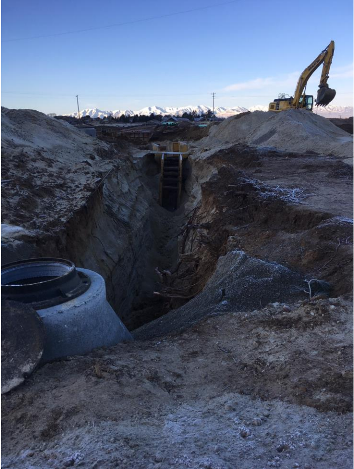
Figure 4 - Earthwork progressing at Gevery
