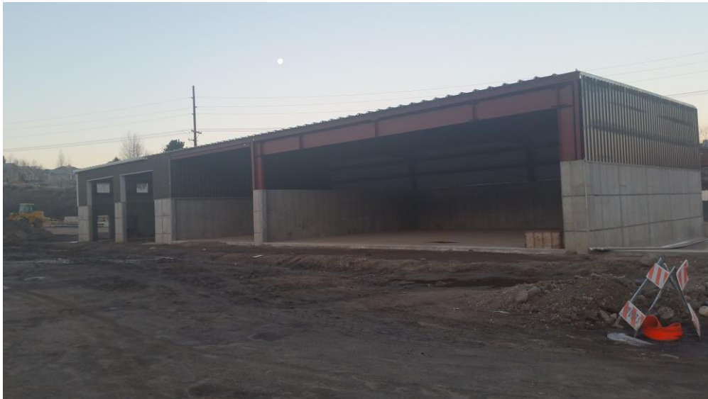
Figure 2 - South face of salt shed. Metal skin almost finished.
