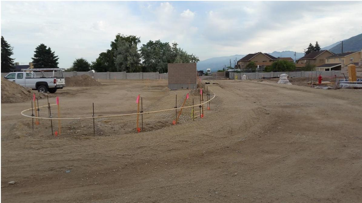
Parking Lot with curb machine stakes and guide rails ready for concrete work
